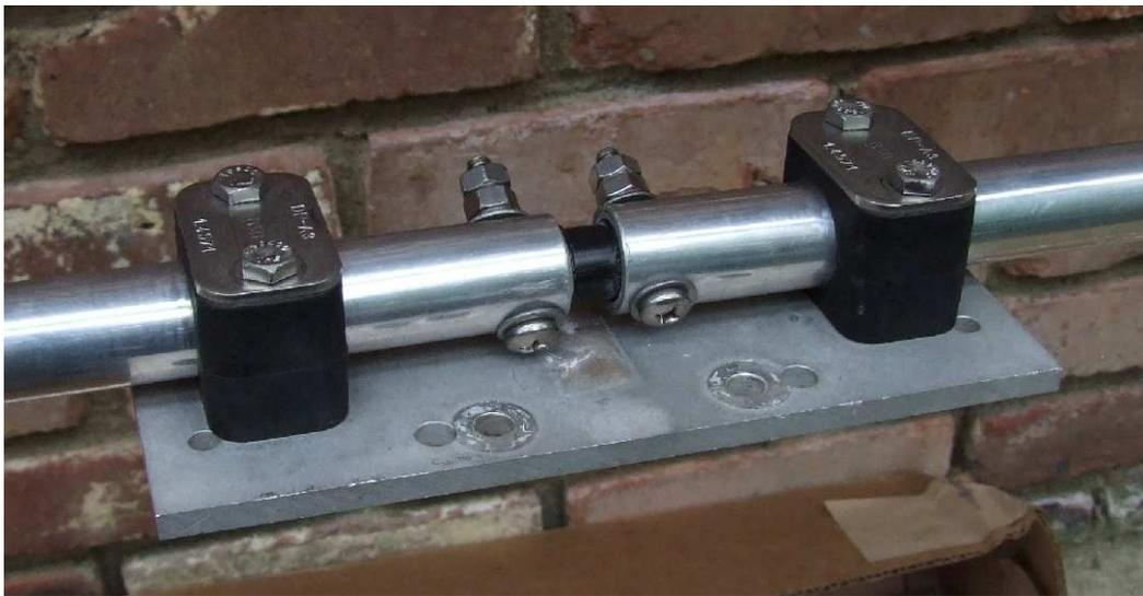
**Figure 12 – Create DE Plate with DE and black plastic insert spacer**
